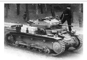
The Pz.Kpfw.II (originally identified as the '2cm MG Panzerwagen') was designed to supplement the Pz.Kpfw.I by providing an automatic weapon capable of firing both a highexplosive and armour-piercing rounds. The KwK.30 (shortened FlaK.30 AA Gun) was used. The initial order for 10-ton panzer was issued in July 1934, and already in October 1935 the first soft steel prototype was tested.
